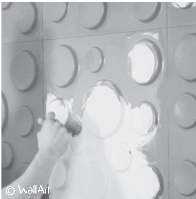
Paint without filling the Joints
