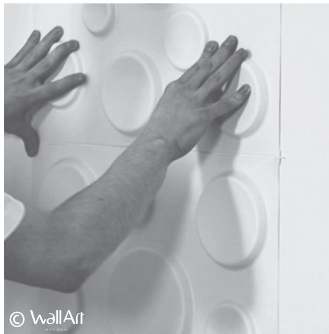
Using Tile Spacers gives best result
